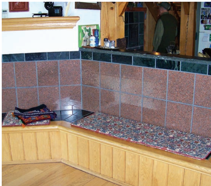
A cozy Old World ambiance and gentle warm radiate from Bill Derrick’s masonry heater. To the left is a Tullikivi soapstone “black oven” cook stove. The hot combustion gases from Bill Derrick’s masonry heater are channeled to create a heated bench in the living room, a big hit on a cold winter day. Photos: Robert Pelletier.
