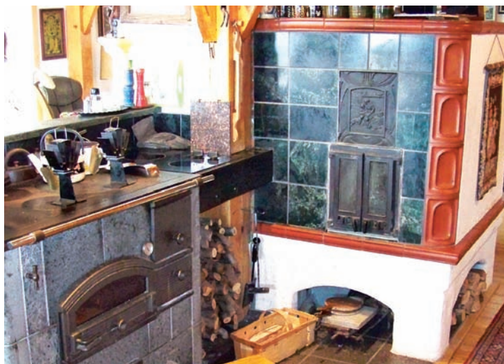
A cozy Old World ambiance and gentle warm radiate from Bill Derrick’s masonry heater. To the left is a Tullikivi soapstone “black oven” cook stove. The hot combustion gases from Bill Derrick’s masonry heater are channeled to create a heated bench in the living room, a big hit on a cold winter day. Photos: Robert Pelletier.
